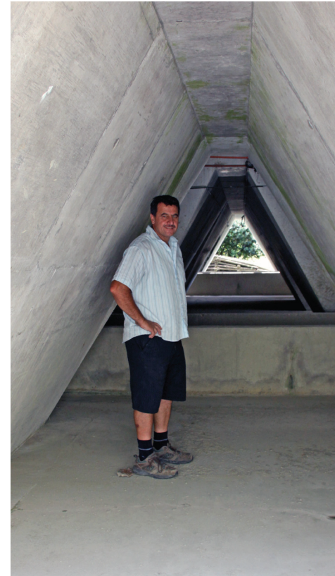
Water Treatment Plant Manager Morgan Goldsmith under the huge sediment tanks.
