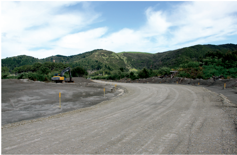
Looking back towards Opoutama from where the new road joins the existing Ormond Drive, it's clear to see work is well on track to have it open before Christmas.
