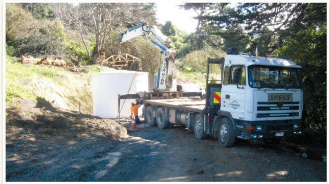
• New tanks go in as part of the Tuai water treatment upgrade.
