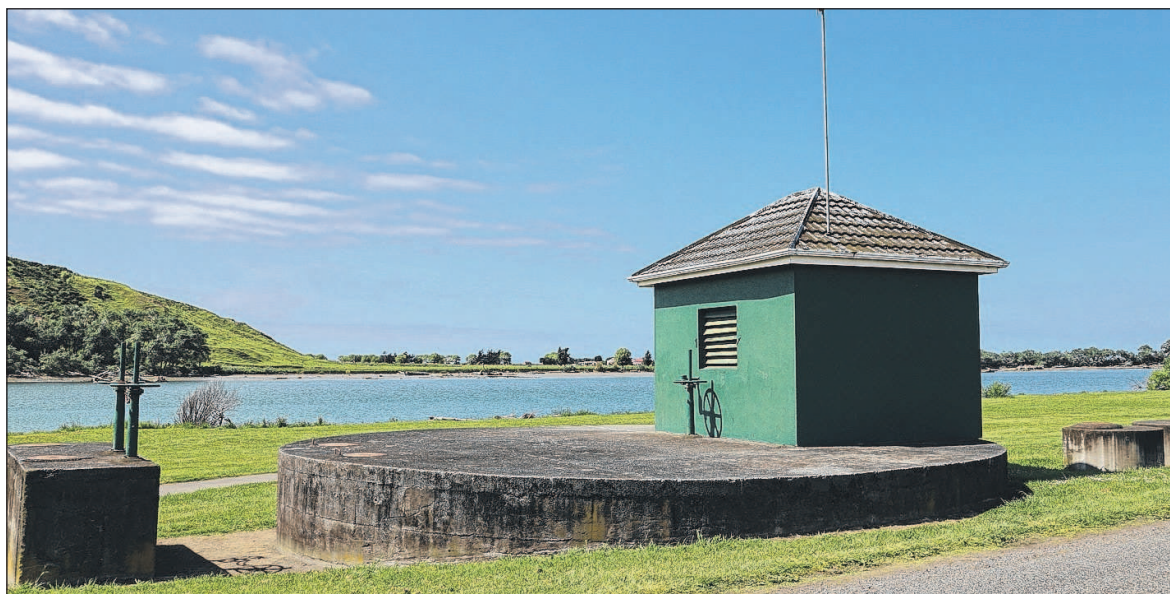
❑ The large Kopu Road pump station.
