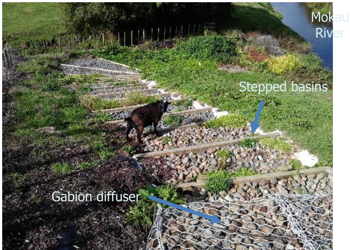
Figure 1: Piopio Cascade Structure
