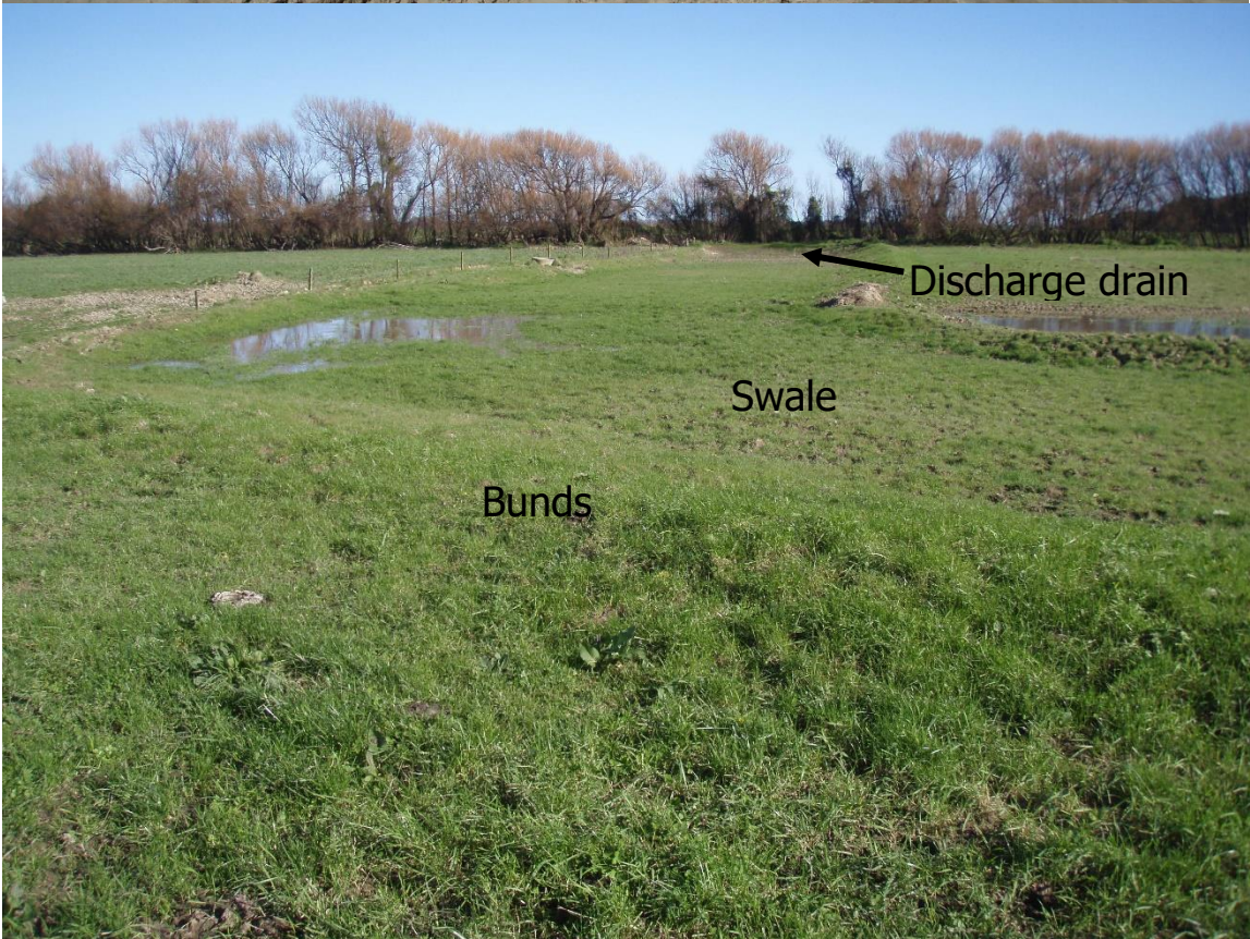
Figure 2: Shannon Vegetated Swale
