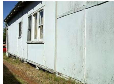
Asbestos Cladding
