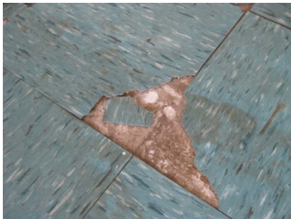
Asbestos Vinyl Flooring
