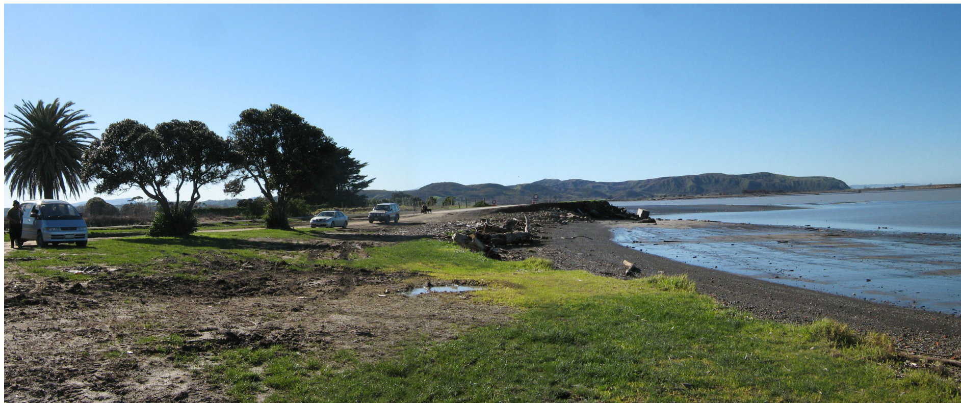
Panorama showing poor condition of car park surfaces in winter
