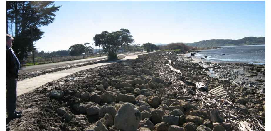
Regional Council erosion protection works 2009
