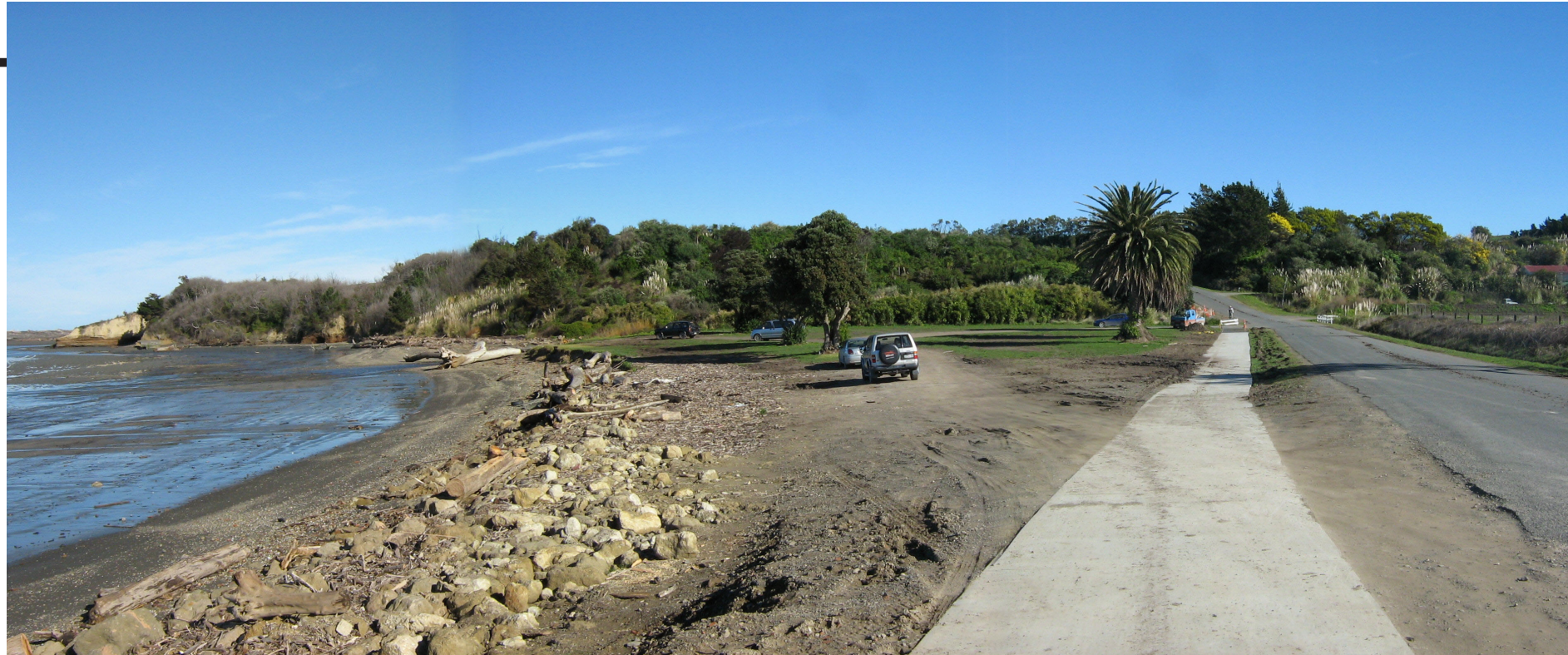
Panorama showing Regional Council shore protection works. Note unsafe intersection of vehicle access to reserve and new walkway
