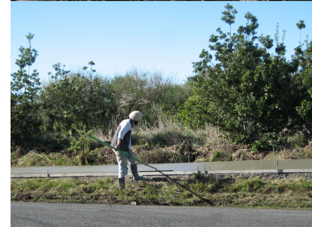
Construction of the Pilot Hill leg of the walkway in 2009
