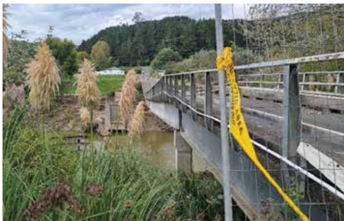
Te Reinga Bridge
