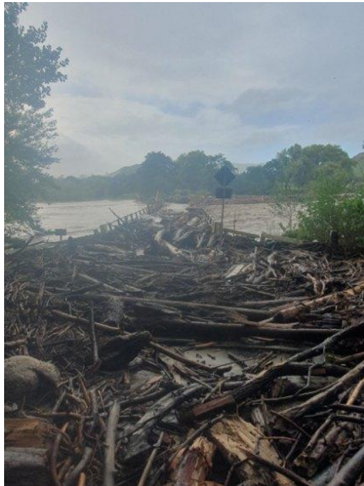
Figure 6. Woody Debris Riverina Bridge, Wairoa River, Marumaru approx 7am February 14, 2023
