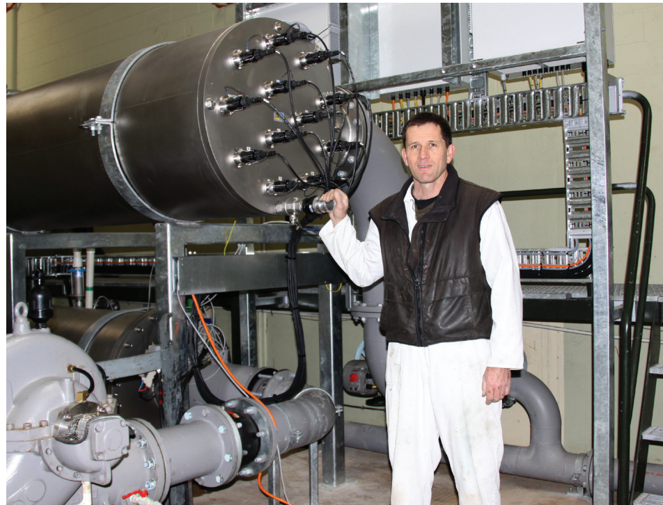
Water Treatment Plant operator Peter Newland checks over one of the new Ultra-Violet reactors that have been installed to provide another measure of ensuring the quality of Wairoa's water supply.
