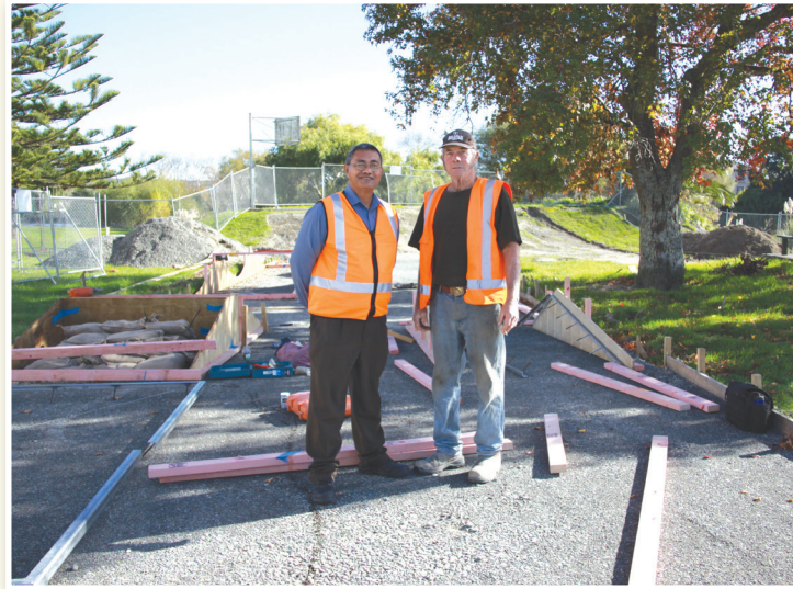
• WDC Project Engineer Pune Brown and QRS Construction Supervisor Chris Baty oversee work on the skatepark extension.
