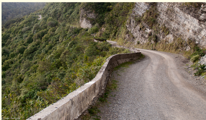
Unsealed section of SH38
